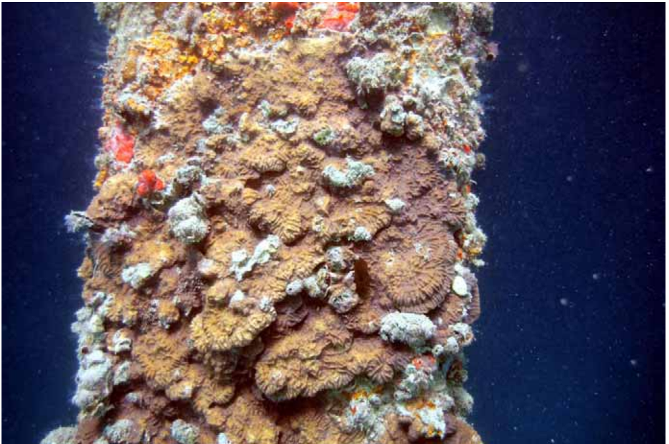
FIGURE 39. SECTOR P-24. Colonies of Leptastrea purpurea (top) and Pavona varians (bottom) on concrete piles on Pier 24 in area proposed for placement of PSI drydock. For location of Sector P-24, see Figure 6.
