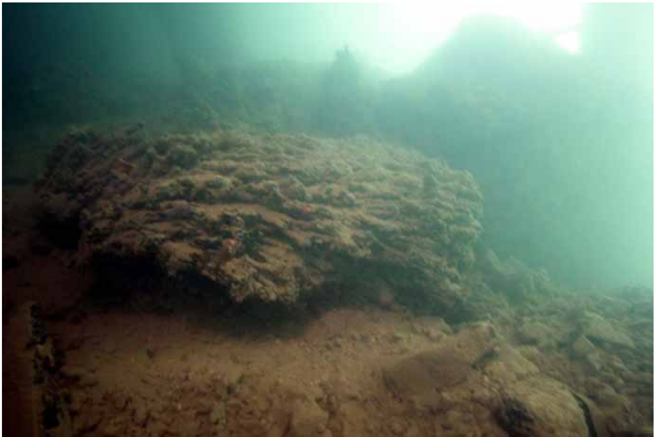
FIGURE 31. SECTOR I. Two photos showing large chunks of calved off sections of old reef that are likely remnants of dredging of Pier 41. For location of Sector I, see Figure 5.
